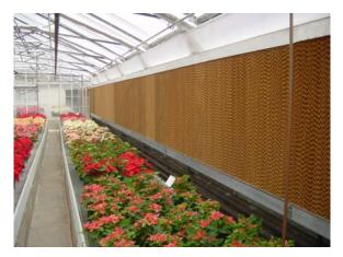
**Figure 20.** Evaporative cooling pad installed along the inside of the ventilation inlet opening. Photo courtesy of A.J. Both, Rutgers University.
