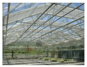
**Figure 19.** Example of an internal shade system in a greenhouse. Photo courtesy of A.J. Both, Rutgers University.
