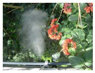
**Figure 21.** Top-down view of a fog nozzle delivering a small-droplet mist for evaporative cooling. Photo courtesy of A.J. Both, Rutgers University.
